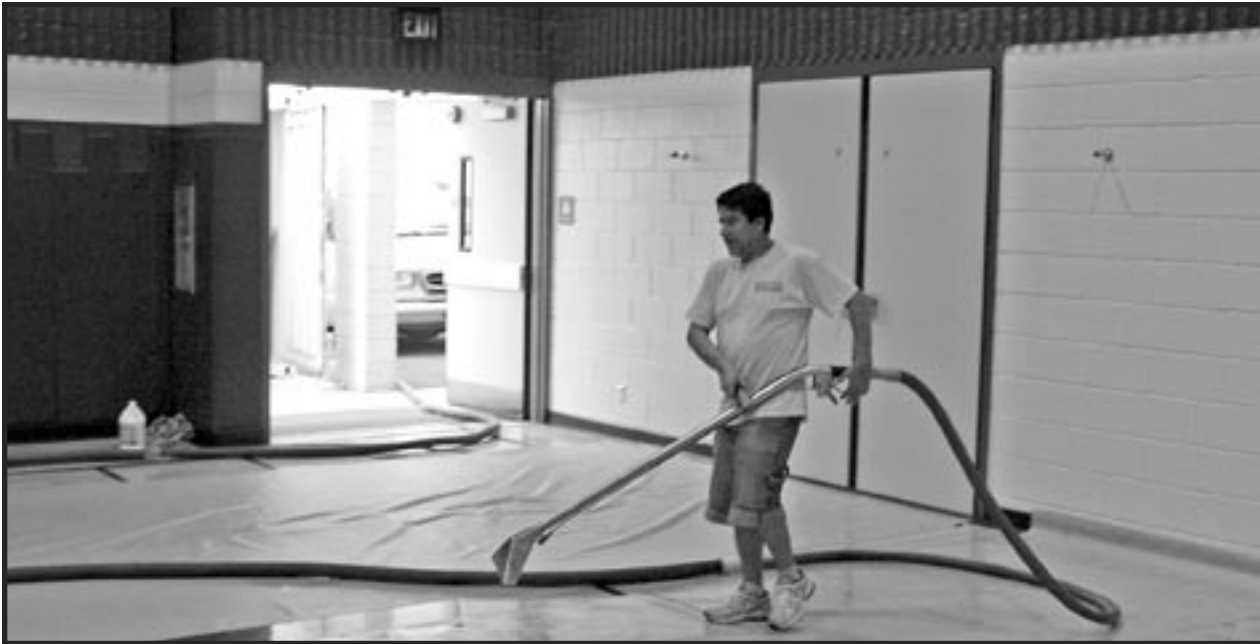
Pedro Victoria of Metropolitan Maintenance Co. cleans gymnasium floor prior to resurfacing.
